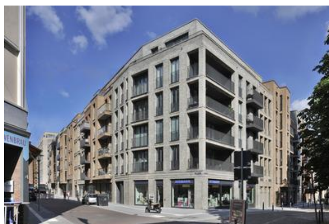
Three derelict buildings were demolished to make room for the new Schlossquartier Kiel. Source: PORR/Arne Biederbeck
