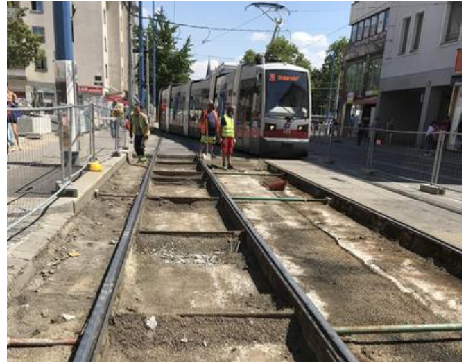
The pre-fabricated concrete slabs and the gravel bed were professionally dismantled. Source: PORR AG
