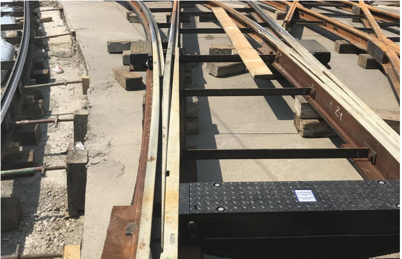
The grooved swivel plates for the intersection were pre-installed. Source: PORR AG
