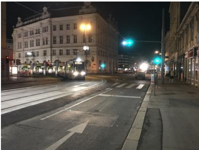
The complete intersection was opened to traffic on the agreed date. Source: PORR AG
