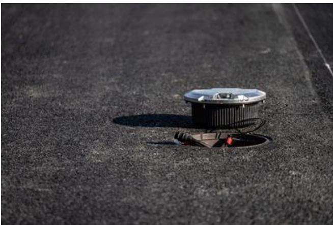
PORR replaced all beaconing lamps on the runway. Source: PORR
