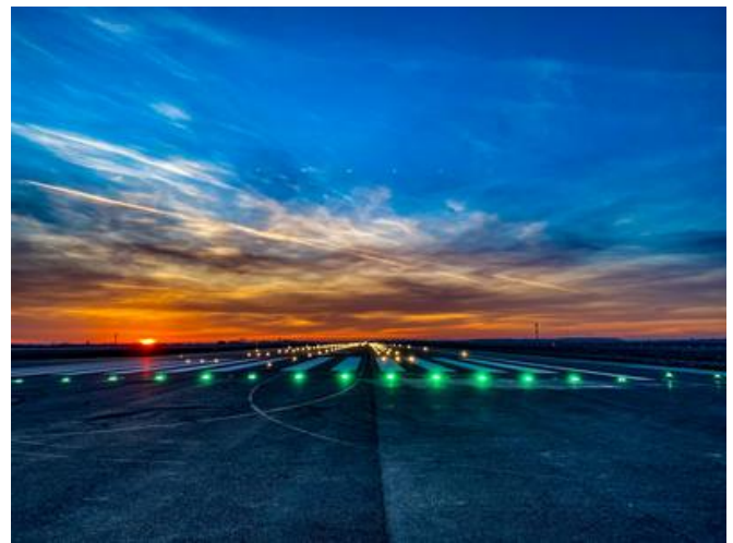
The newly installed beacons illuminate the finished runway. Source: PORR
