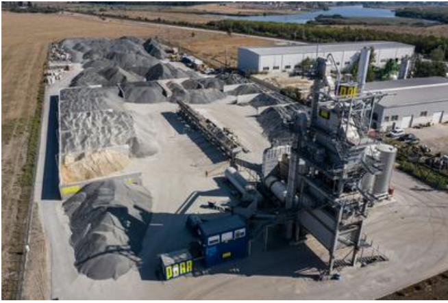
PORR's in-house asphalt plant in Bucharest produced most of the asphalt needed for the runway project. Source: PORR
