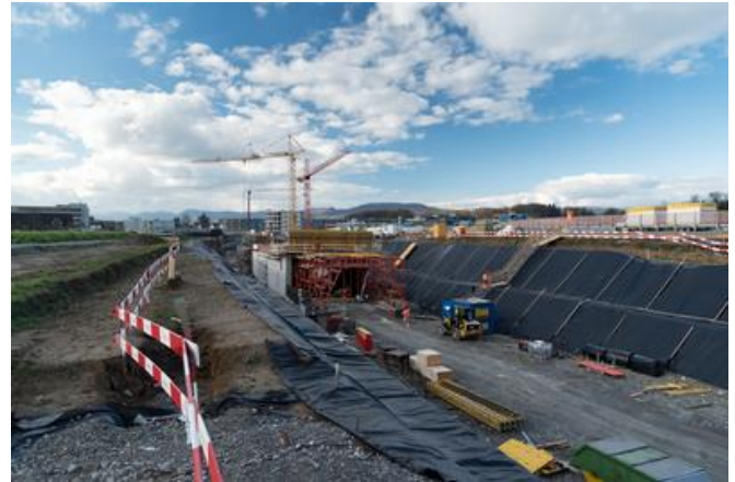
Start of the first stage of concreting the tunnel ceiling and tunnel entrance with formwork and curing carriages. Source: PORR
