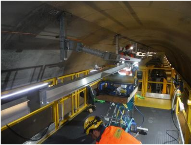
A special procedure was developed for the installation of the overhead conductor elements. Source: CPC/Petzold
