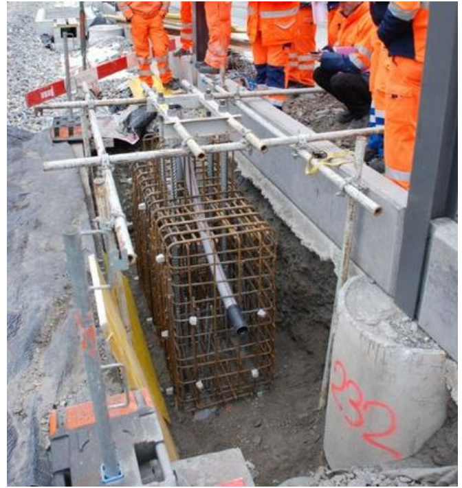
The foundation work for the catenary supports on the track outside the tunnel became a real challenge, because the planning basis for the project did not match the conditions on site. Source: CPC/Chladek
