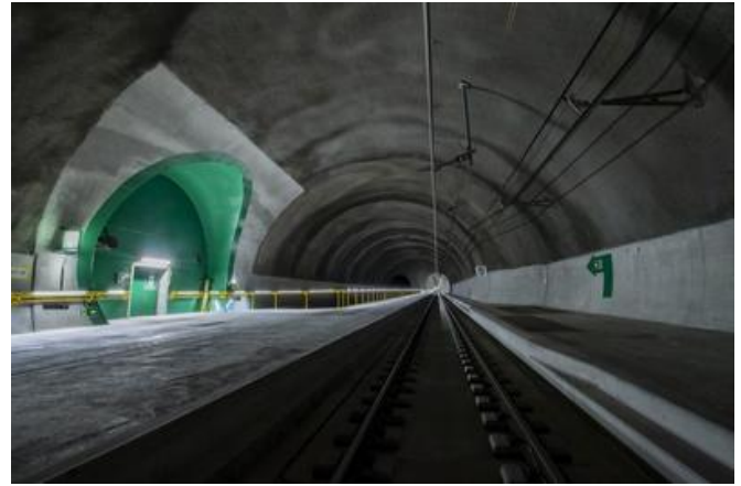
From December 2020, passenger trains will pass through the Ceneri Base Tunnel at speeds of up to 250km/h. Source: AlpTransit Gotthard AG
