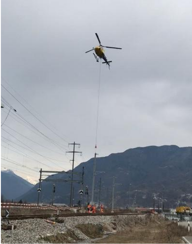
The catenary supports outside the tunnel were positioned from a helicopter. Source: CPC/Petzold
