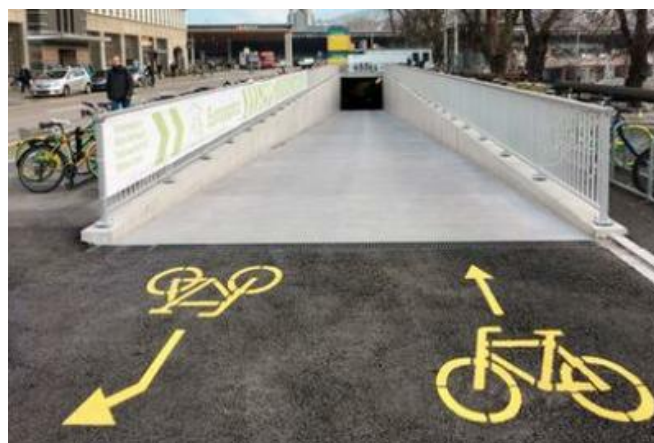
Entrance and exit to the bicycle garage. Source: PORR
