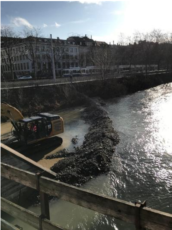
In order to allow the dismantling process to be carried out seamlessly, floodable embankments were created to expose the riverbed beneath individual spans. Source: PORR
