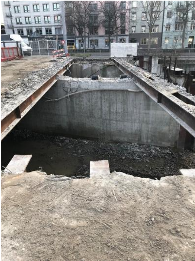
Around 380t of steel was removed when the old Postbrücke was dismantled. Source: PORR
