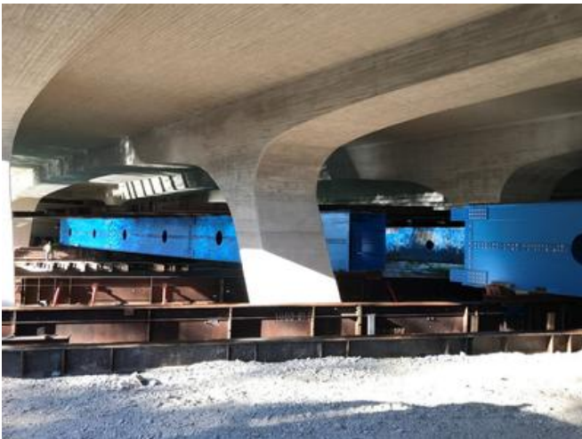
View under the new bridge while moving the scaffolding. Source: PORR
