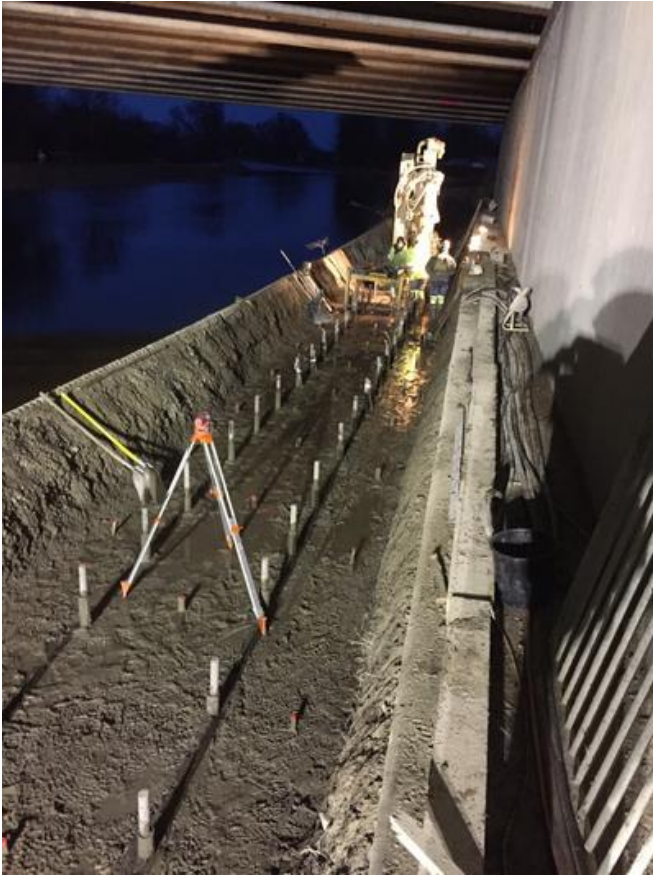
The small bored piles for the skidways were constructed by PORR Grundbau. Source: PORR
