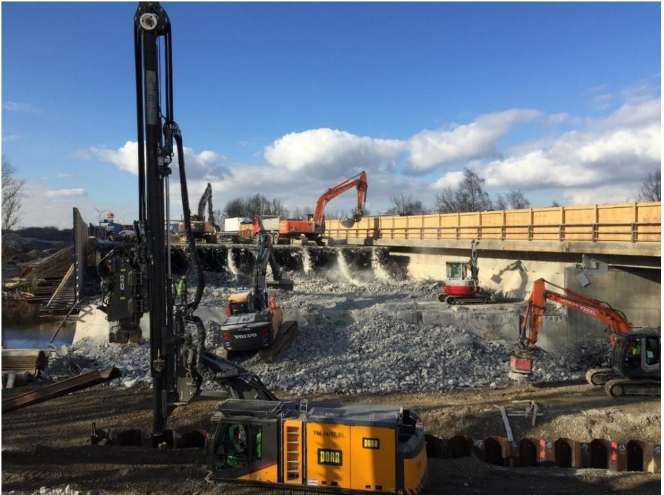
The existing superstructure is being demolished in the background, while the sheet piling work for the new construction is being carried out in the foreground. Source: PORR
