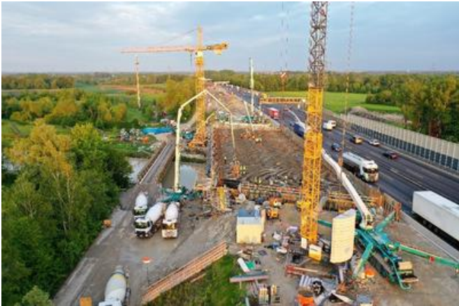
The delivery of concrete for concreting the superstructure proved to be a real challenge because of the high volume of traffic. Source: PORR
