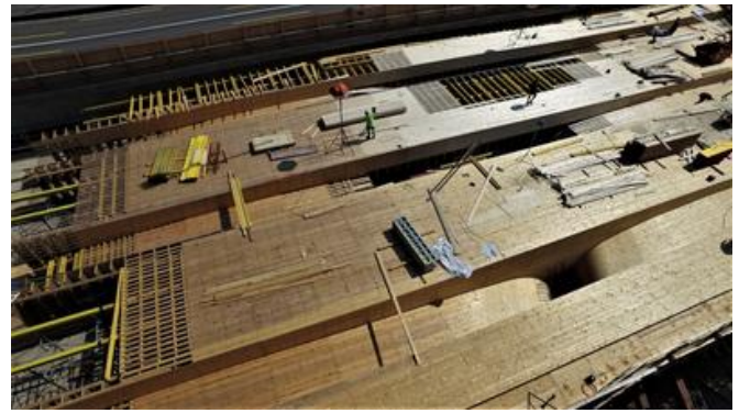
The load-bearing formwork was constructed with parabolic longitudinal girders and conical piers. Source: PORR
