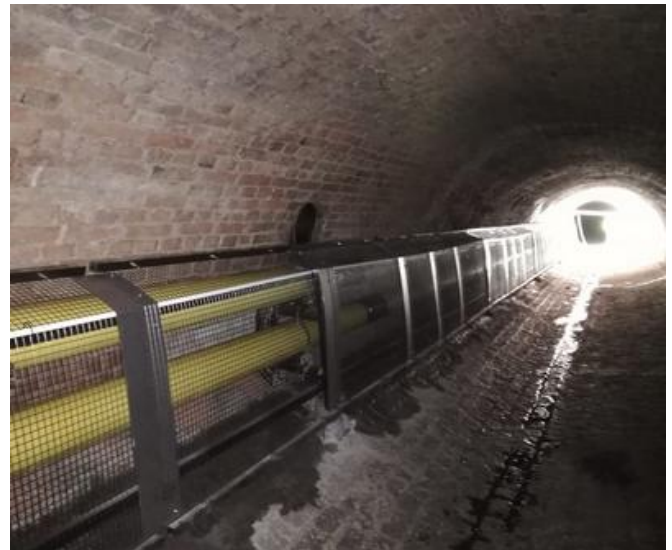
The completed steel pipeline in the Krottenbachkanal sewer, enclosed with a stainless steel grid construction. Source: PORR
