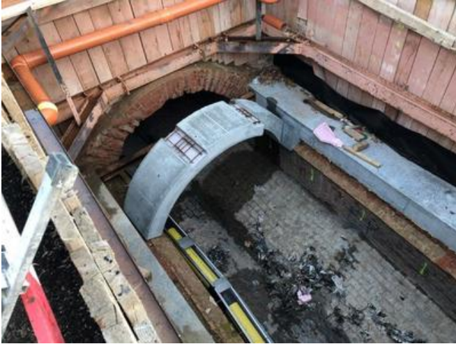
Positioning the precast concrete elements to close the brick vault of the Krottenbachkanal. Source: PORR
