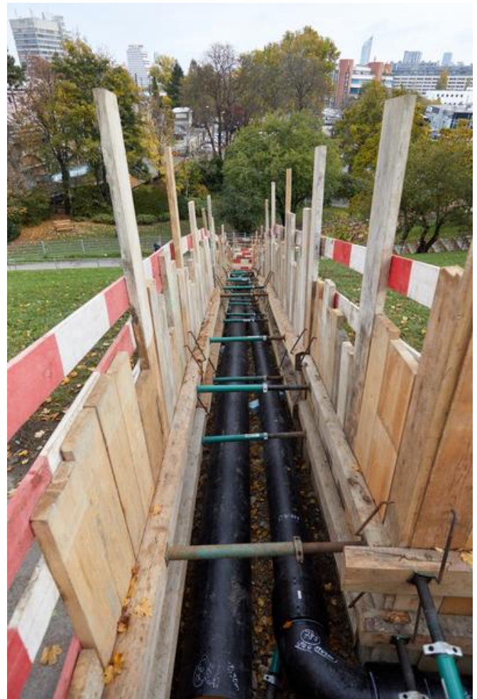
The newly laid district cooling pipeline with a view of the Wertheimsteinpark. Source: PORR
