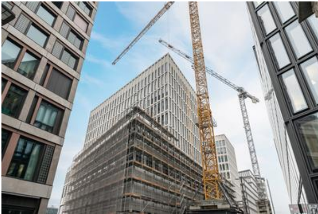
The façade comprises double-leaf, closed aluminium-profile window elements, with freely adjustable curtains in the space between the panes. Source: PORR
