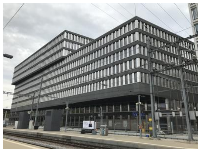
A large, cantilevered section was constructed above the first floor, with loads from the eight floors above applied to this section. Source: PORR
