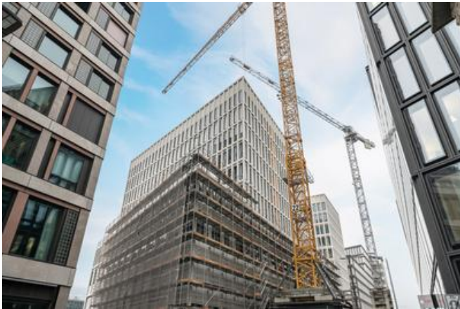
The façade comprises double-leaf, closed aluminium-profile window elements, with freely adjustable curtains in the space between the panes. Source: PORR
