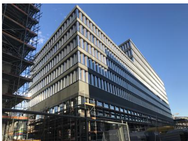
The building on site B was realised as a reinforced concrete skeleton construction. Source: PORR
