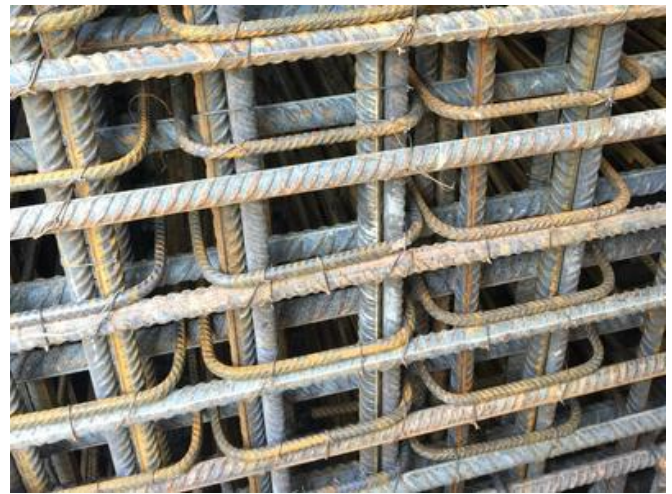
The complexity of the frame and the jointless construction resulted in a complicated reinforcement layout with very high reinforcement density of the individual components. Source: PORR
