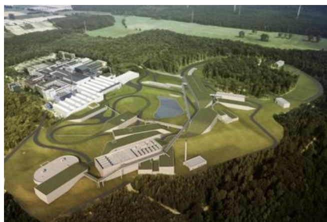
The new particle accelerator centre is to be built on a 20ha site by 2025. Source: ion42/FAIR
