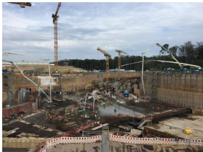
PORR will carry out over 100 large-scale concreting operations averaging 1,500m 3 of concrete throughout the duration of the project. Source: PORR
