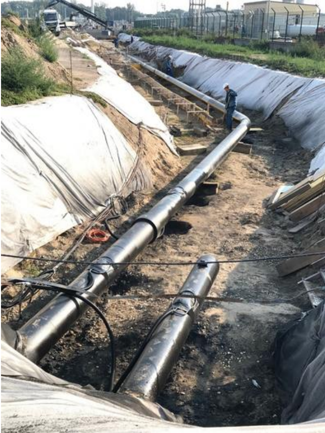
The damaged pipeline had to be excavated along a length of 140m in preparation for replacement. Source: PORR
