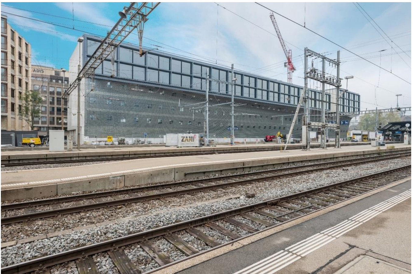
The eye-catching glass brick façade at the Zurich's central station, with its multiple curves, represents a technological milestone for PORR. Source: PORR
