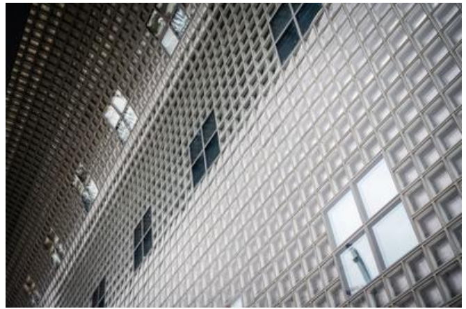
A view of the glass brick façade from below, looking upwards. Source: PORR
