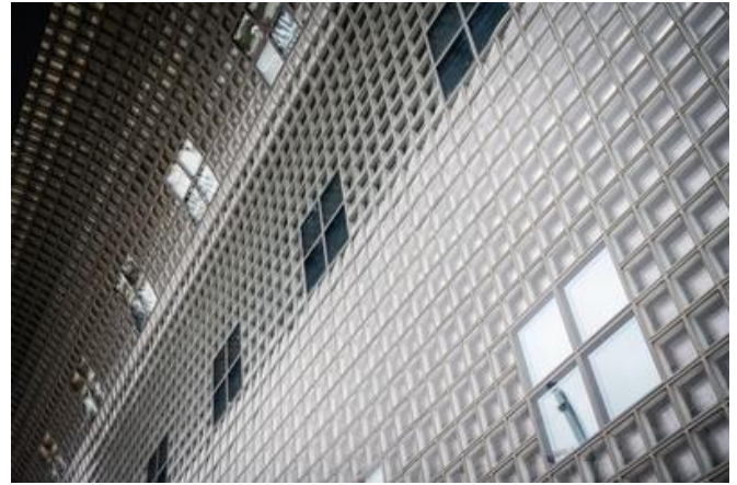
A view of the glass brick façade from below, looking upwards. Source: PORR
