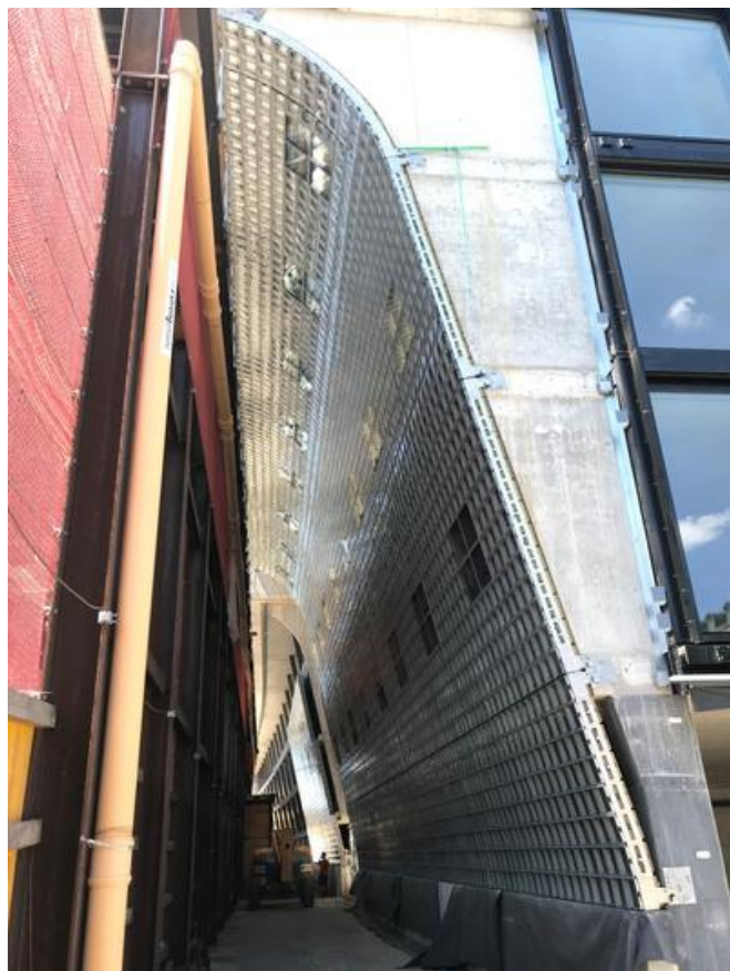
This side view shows the high geometric complexity of the glass brick façade. Source: PORR
