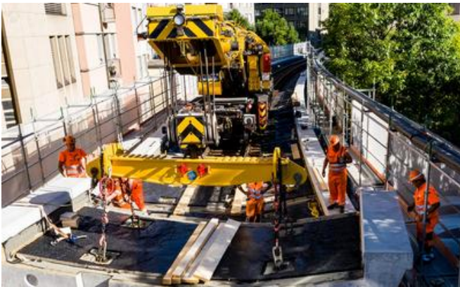
A new railbed with concrete elements was rerouted over an existing viaduct. Source: PORR
