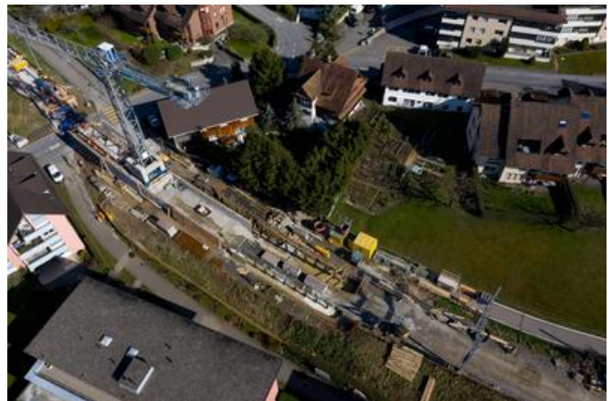
The extremely cramped conditions presented major logistical challenges. Source: PORR
