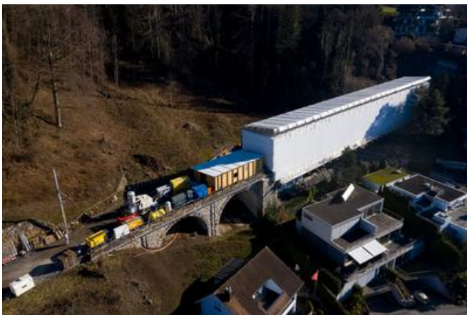
The steel bridges had to be encased for the corrosion protection work. Source: PORR
