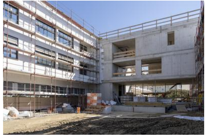
For maximum efficiency, parallel teams worked on the north and south tract on staggered construction stages. Source: PORR
