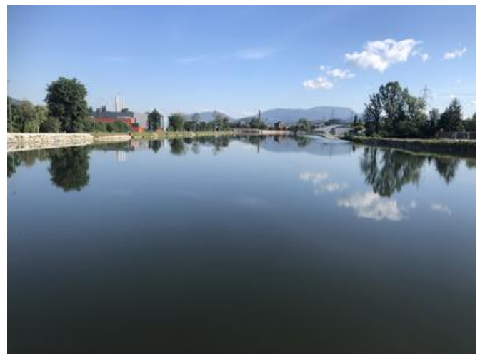
Enough water behind the new Mur dam to supply the energy requirements of 45,000 people. Source: PORR
