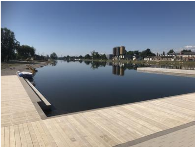
The shallow water zone with boat moorings and "Am Grünager" rowing area. Source: PORR
