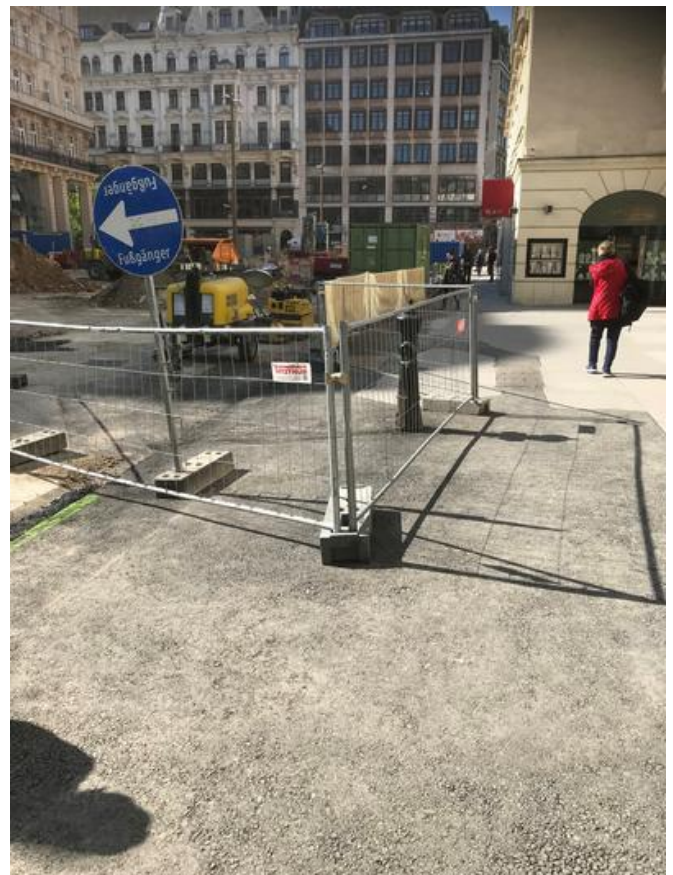
Over 1,000m of temporary fencing was erected. Source: PORR
