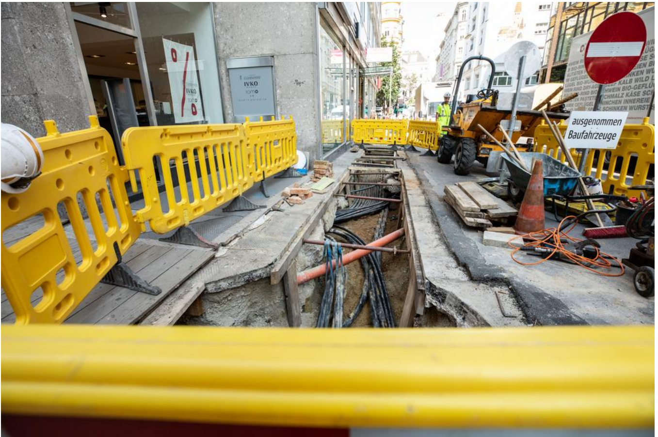
The cramped conditions around the construction area presented various challenges for the WIBEBA team. Source: PORR
