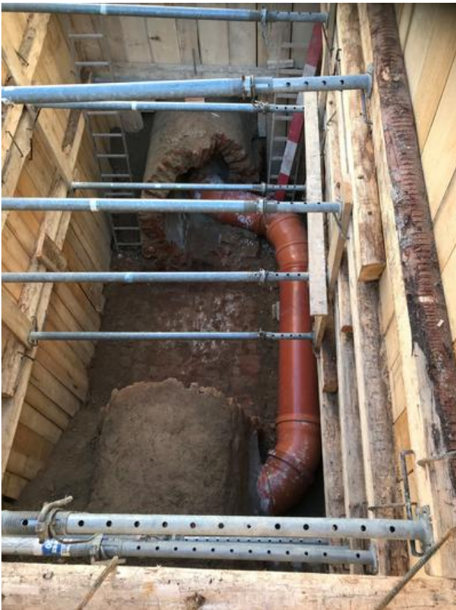
A specially built bypass ensured the sewage system continued to operate. Source: PORR
