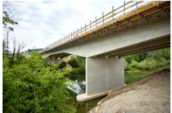
The consortium is building 14 of the 17 new bridges on the new route. As well as a number of smaller structures, these include the north and south bridges over the River Erlauf. Source: PORR
