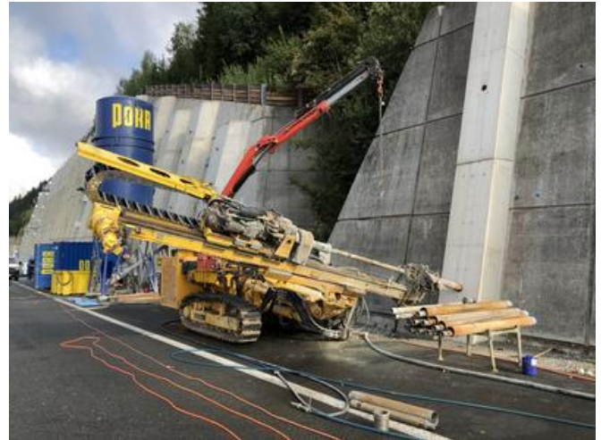
The drill holes in the lower level were drilled using a crawler drill rig. Source: PORR Specialist civil engineering
