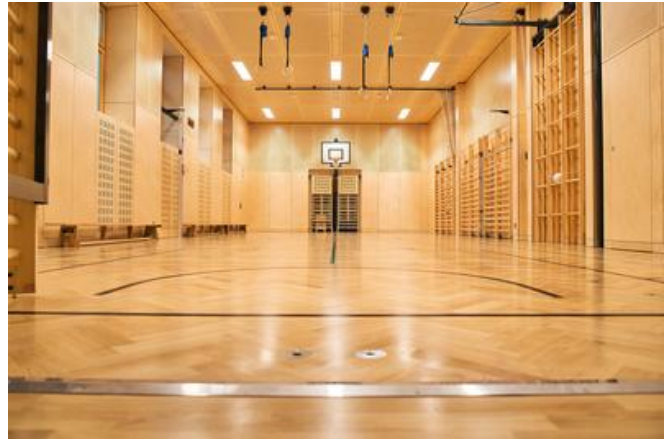
The sports hall on the first floor was completely gutted and rebuilt by PORR. Source: PORR/Philip Trummert
