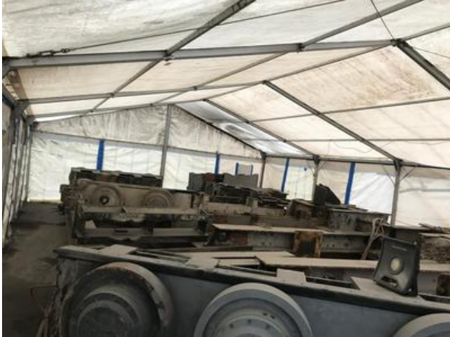
The team worked in a dust-tight treatment tent to strip the steel parts. Source: PORR
