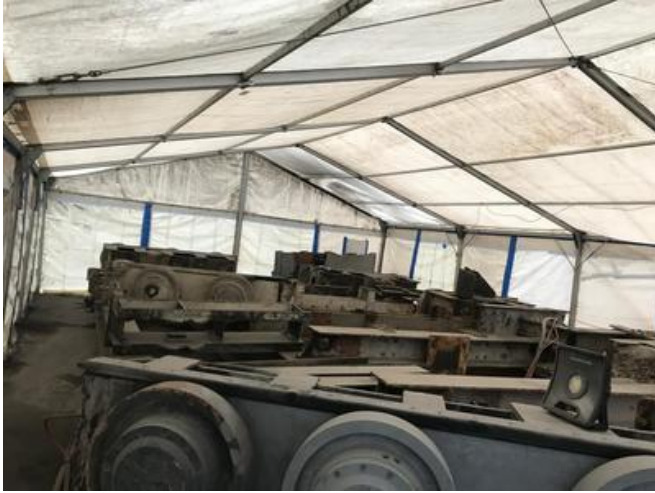
The team worked in a dust-tight treatment tent to strip the steel parts. Source: PORR
