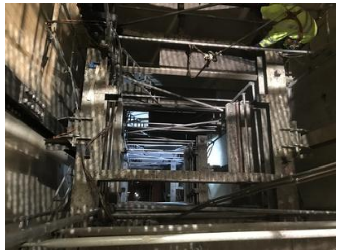
PORR built a 560 m 3 interior scaffold for safe removal of the steel parts. Source: PORR
