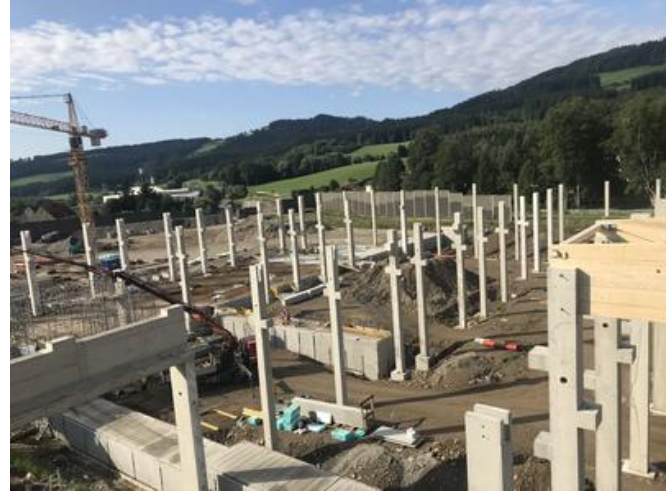
PORR carried out the surveying work for the 144 footings and columns itself. Source: PORR
