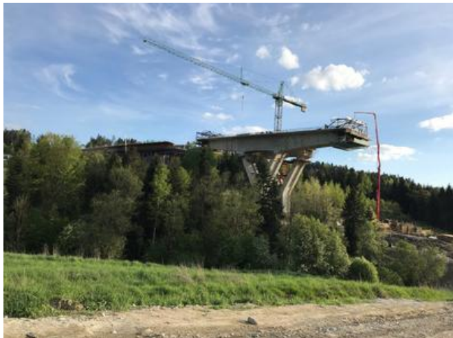
The bridge is about 50m high at its highest point. Source: PORR
