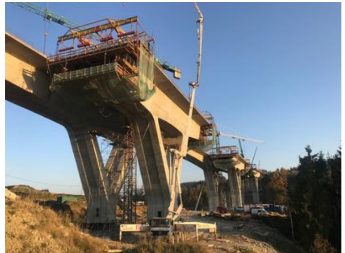
Sliding devices were used to concrete the individual bridge segments. Source: PORR
