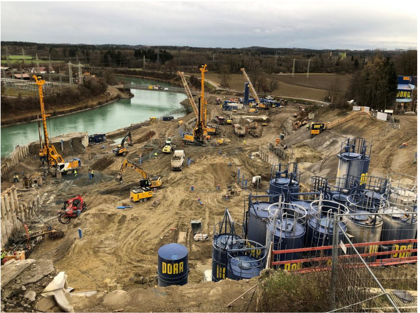
During creation of the construction pit for the Töging power station consortium, PORR impressed its employers with numerous optimisations to the original plans. Source: Thomas Wiczorek
