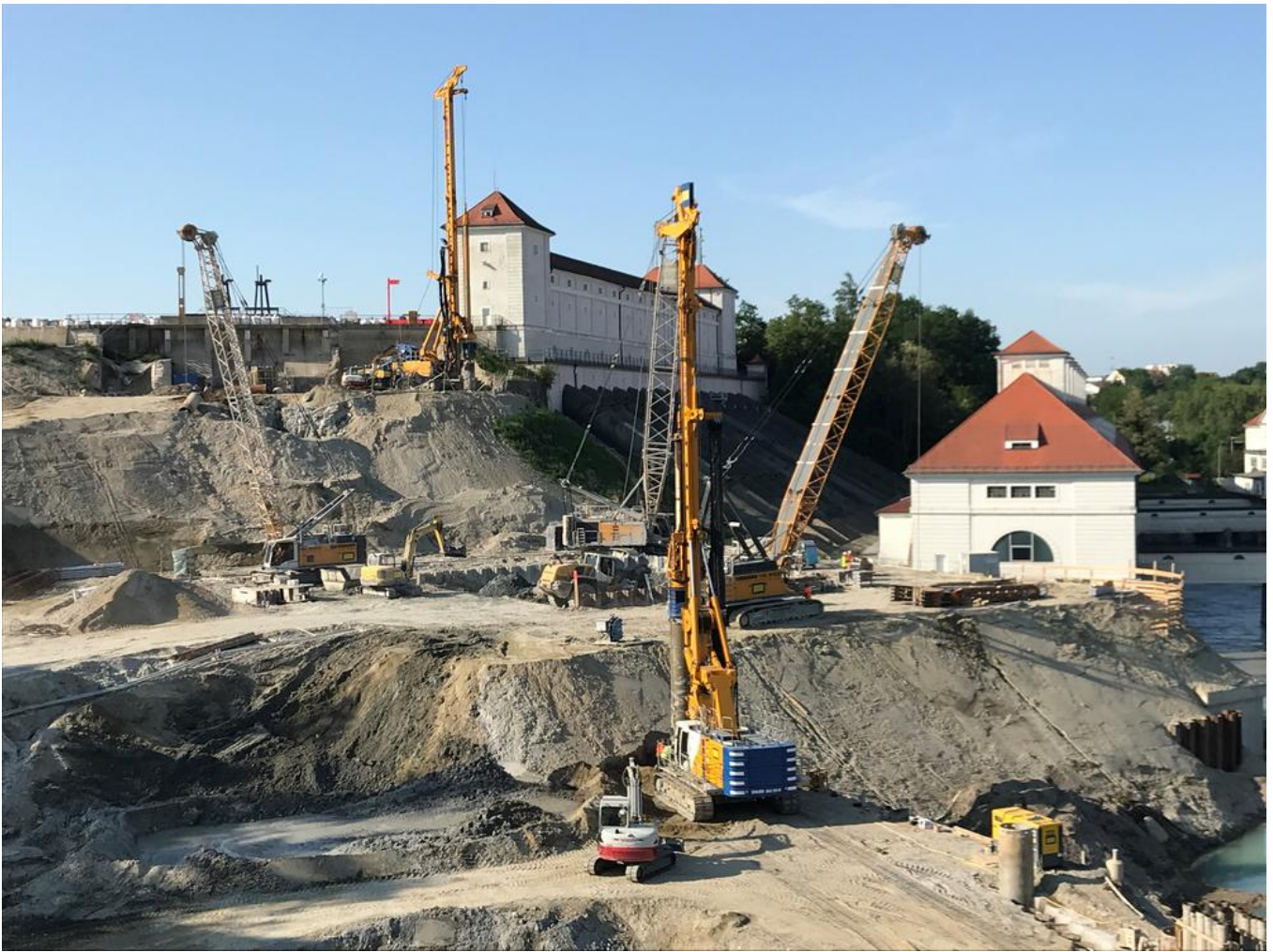
Creating the main construction pit involved almost every type of work in the specialist civil engineering department. Source: Markus Trinkl
