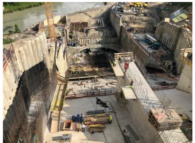
The base slab is nearly complete. Source: Thomas Wiczorek
