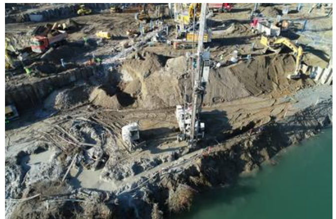
The execution variant PORR designed for the construction pit was tested in advance for feasibility in a large-scale test in Himberg. Source: Markus Trinkl
