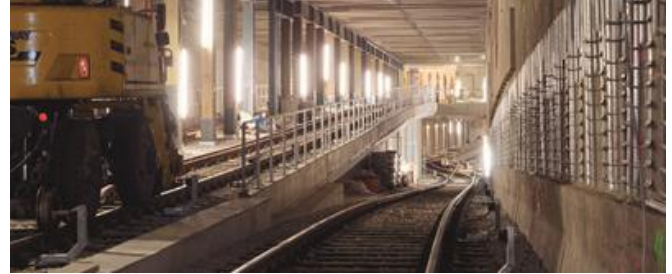
A view into the renovated tunnel, showing the track installation. Source: PRGU5
