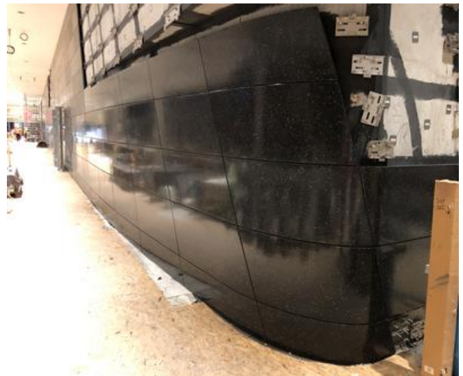
Every façade slab is slotted into its allocated place like a jigsaw piece. Source: PORR/Ilmert
