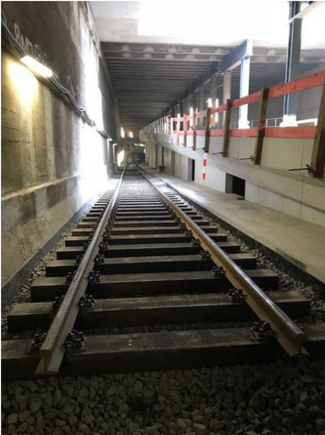
Altogether, the consortium installed some 2,000m of track and 14 switches. Source: PORR/Abraham
