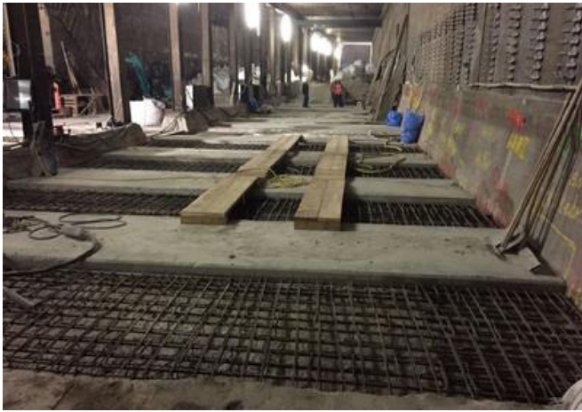
The tunnel renovation was carried out using a back-and-forth process in sections 1.5m wide. Source: PORR/Abraham
