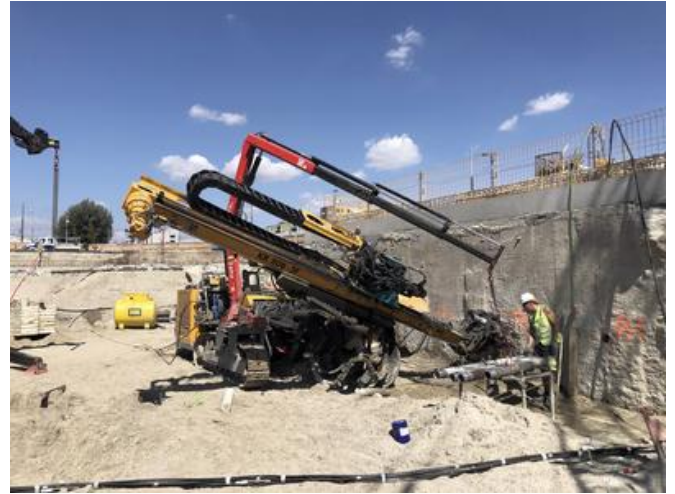
The diaphragm wall was anchored with 183 temporary anchors. Source: PORR
