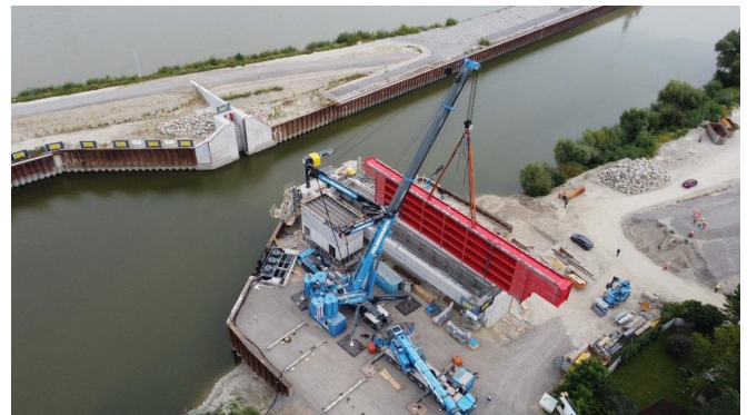
Lifting the upper part of the port gate, weighing around 130 tonnes. (c) Kavin Ofner, Andritz Hydro GmbH
