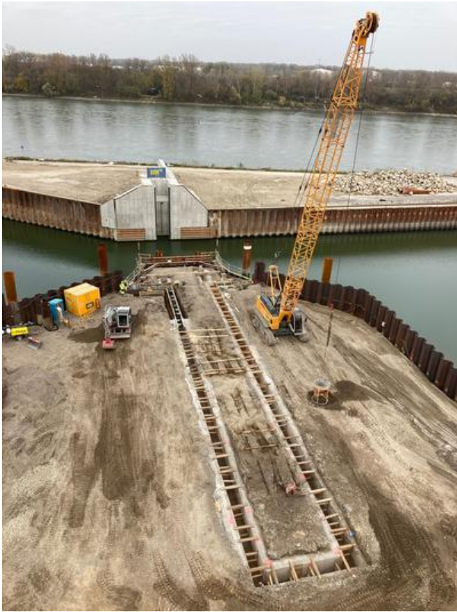
Preparations for work on the diaphragm wall in construction phase 2. (c) PORR
