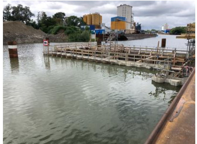
The sheet piling enclosures during construction phase, under flood conditions. (c) PORR
