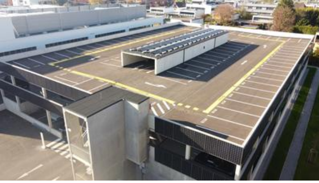
With a multi-storey car park on three levels and an expansion of the existing underground garage, the BMW site in Salzburg now offers more than 470 parking spaces. (c) PORR
