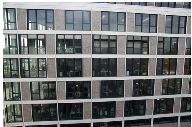
Façade view Image: PORR AG
