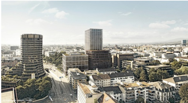
A glimpse of the future: This is how Baloise Park in Basel will look by the end of 2019. PORR SUISSE is building the head-quarters (left) and office building with training center (right). Image: Basler Versicherung
