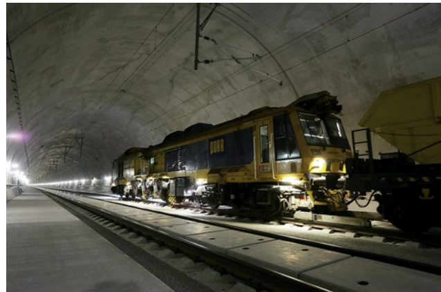
Accessibility for emergency vehicles with a guide rail function is a new development of the PORR slab track system. Image: PORR AG
