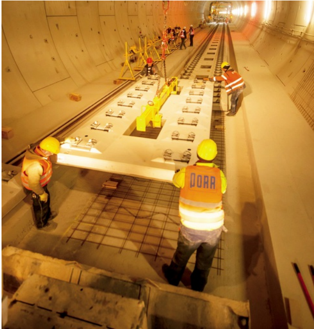
Installation of the PORR slabs in tight areas. Image: PORR AG
