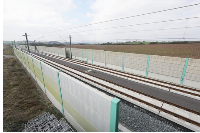
PORR's Slab Track Austria system was implemented on a total of three sections of the new VDE 8 high-speed line. Image: PORR AG
