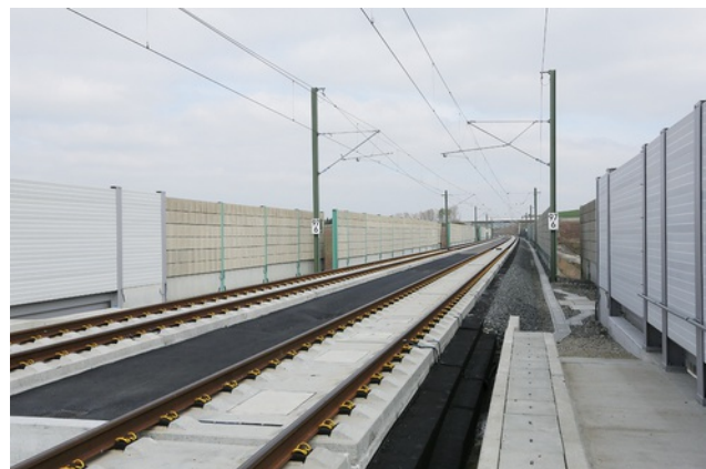
PORR was also commissioned to design and build noise and wind protection barriers for the operating speed of up to 300 km/h. Image: PORR AG
