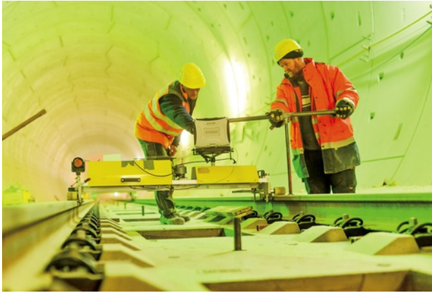
The high degree of prefabrication in the factory allows quick installation and little rework on site. Image: PORR AG
