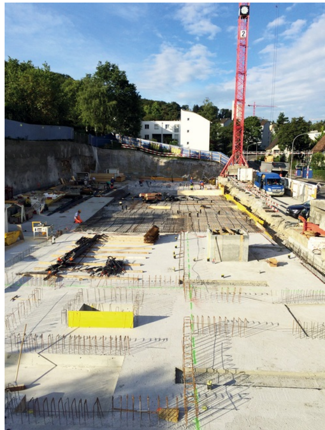
Construction pit Image: PORR AG
