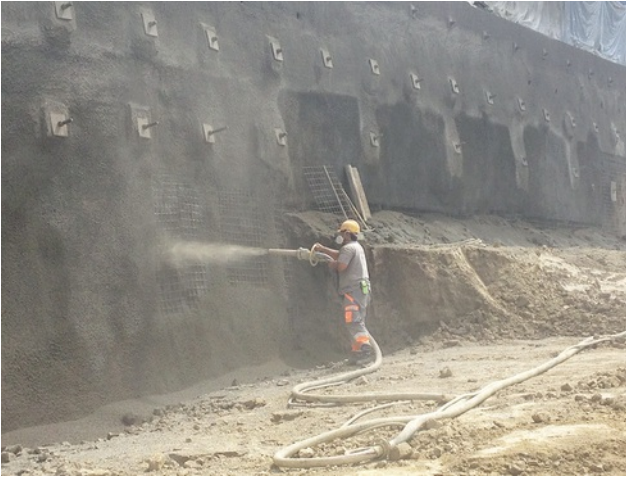
Nail wall Image: PORR AG
