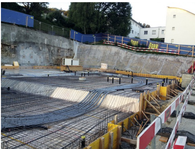
Geothermal probes in the floor panel Image: PORR AG
