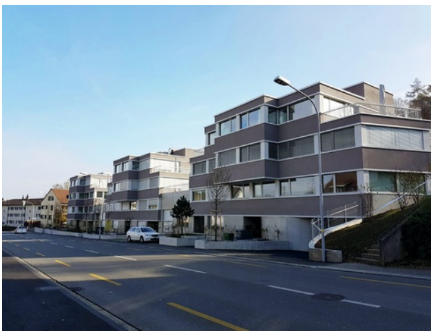
View from a north-westerly direction Image: PORR AG
