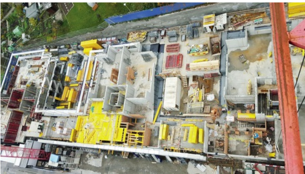
Ground floor carcass floor Image: PORR AG
