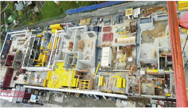
Ground floor, carcass Image: PORR AG
