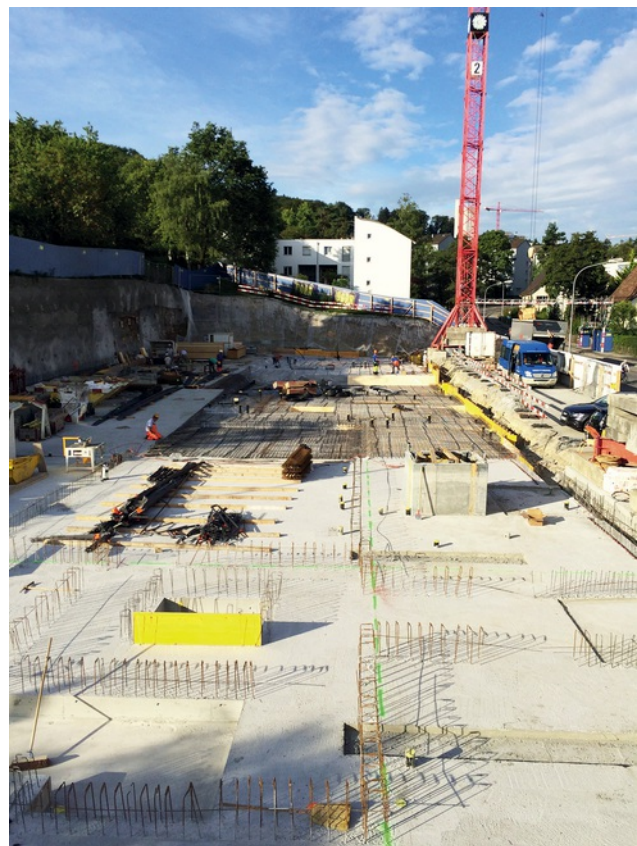
Construction pit Image: PORR AG
