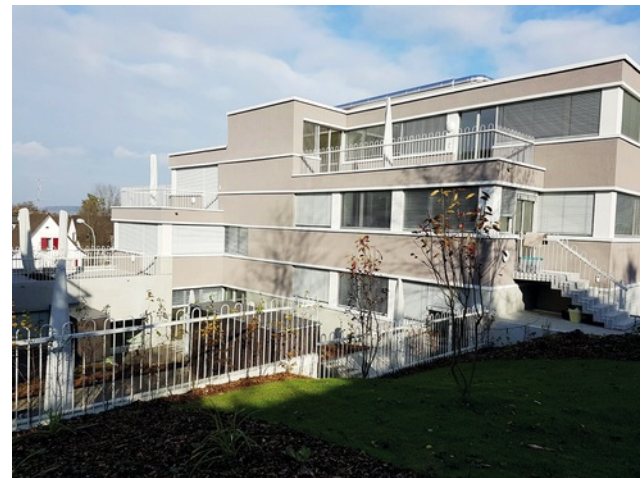
View of the building B facade / garden side Image: PORR AG
