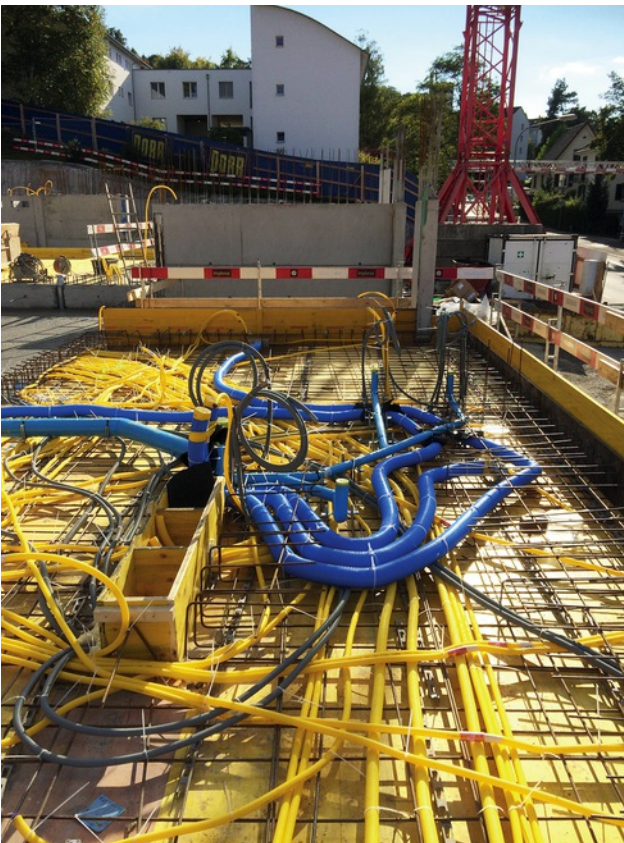
Ceiling inlays above the ground Image: PORR AG
