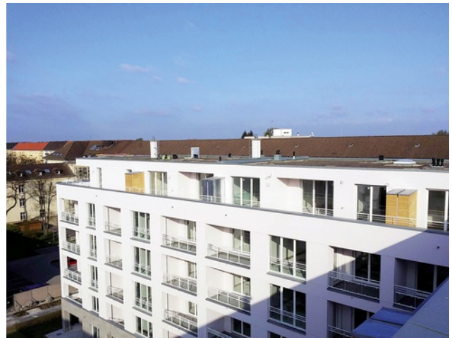
Façade of structure A, courtyard side Image: PORR AG
