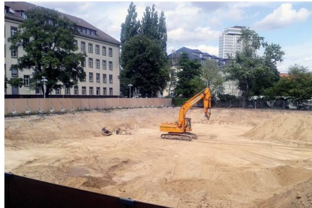
Construction pit of structure A Image: PORR AG
