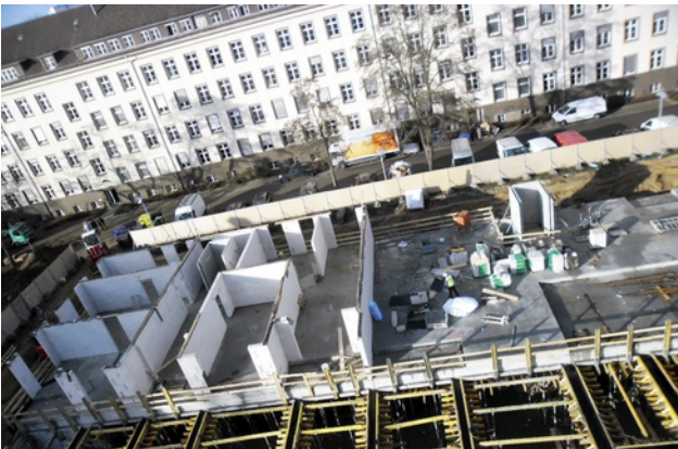
Ground floor carcass, structure A Image: PORR AG
