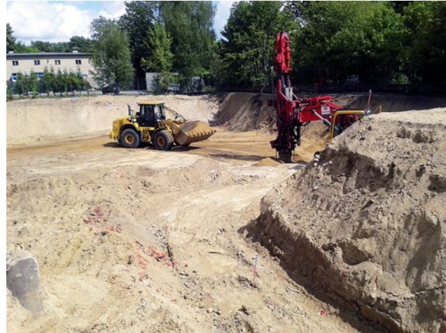
Construction pit of structures A and B Image: PORR AG
