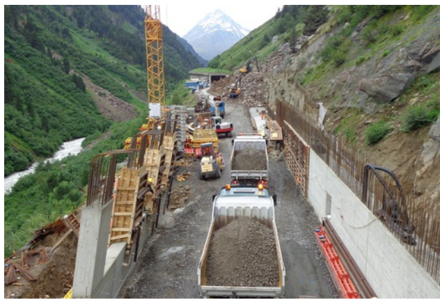
Downhill wall columns Image: PORR AG
