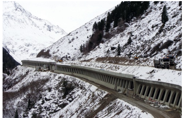
State of construction November 2013 Image: PORR AG
