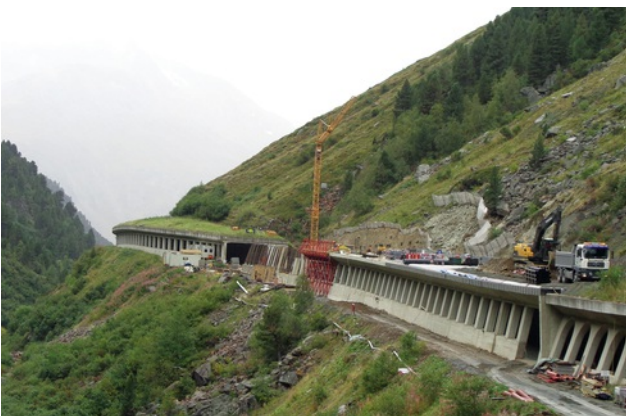
State of construction September 2013 Image: PORR AG
