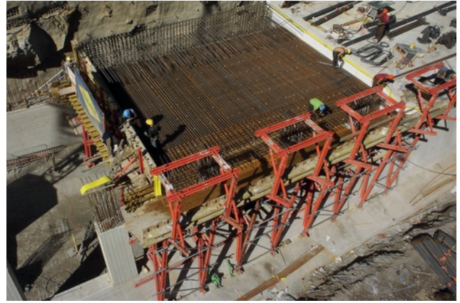
Laying of reinforcements at frame superstructure Image: PORR AG
