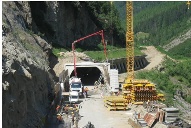
Uphill strip foundations Image: PORR AG
