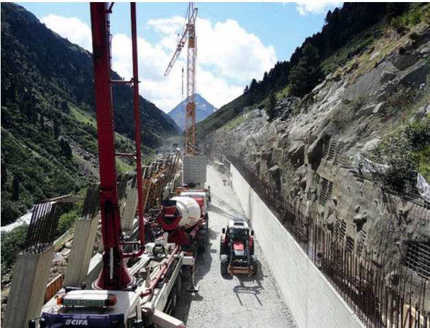
Keeping the road open for traffic Image: PORR AG
