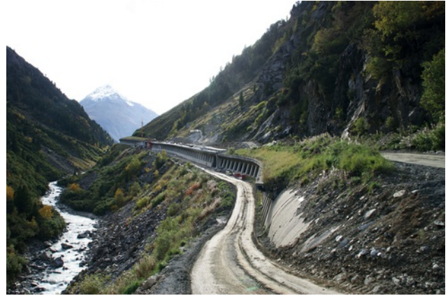
Access road to intermediate dumping area Image: PORR AG
