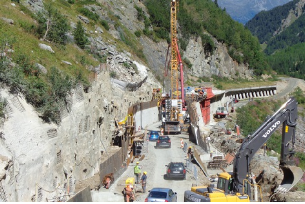
Keeping the road open for traffic Image: PORR AG
