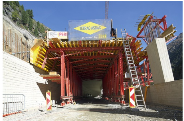
Gallery form work carriage Image: PORR AG
