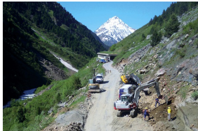
Rock stabilisation and excavation work Image: PORR AG
