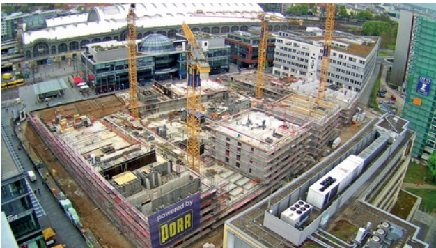
Building shell Image: PORR AG
