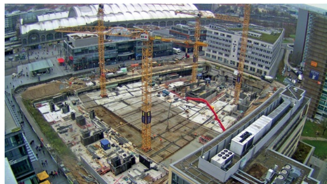
Floor slab 2 basement storey Image: PORR AG
