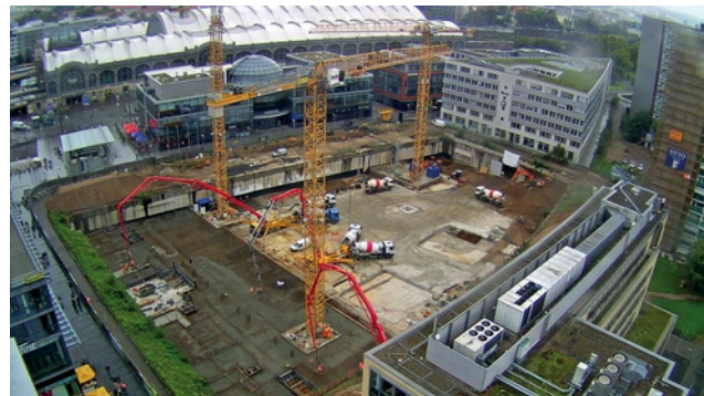
Bottom slab Image: PORR AG
