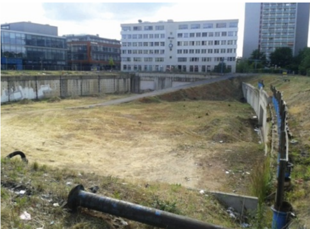
Construction pit Image: PORR AG
